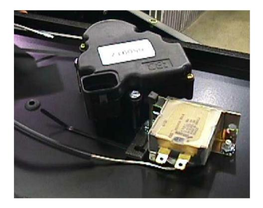
If freeze switch fails closed, compressor runs all the time and never cycles – evaporator eventually freezes up
