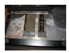
Mark and drill pilot holes for 4 mounting feet. The unit has 8 possible locations but you will only use 4. Use locations as indicated in the photo.
